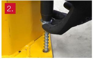
2. Drive in Concrete Screw with Filling Washer until the anchorage depth  $\mathbf{h}_{\mathrm{nom}}$  is reached
