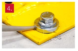
4. Fill the annular gap between Concrete Screw and fixture through the hole of the Filling Washer until resin leaks out.
