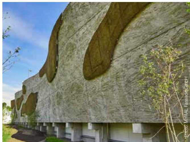
Noise protection wall of the Krombacher brewery in the form of moss islands on an area of 270 square meters
